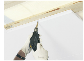
Focus F is installed by screw fixing
