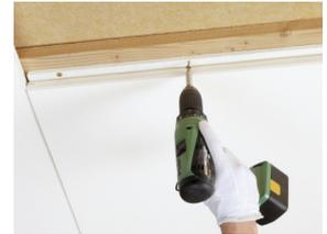
Master F is installed by screw fixing
